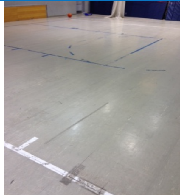
Hope School Multi-Purpose Room Floor
