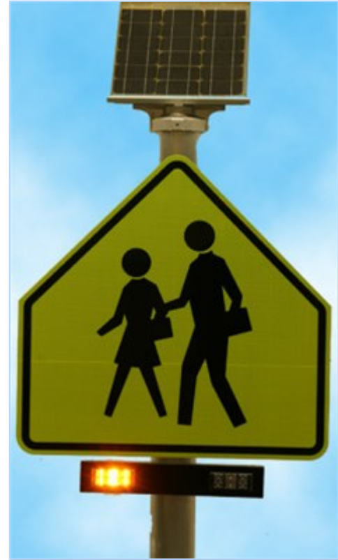
Figure 3-2 – Rectangular Rapid Flash Beacon
