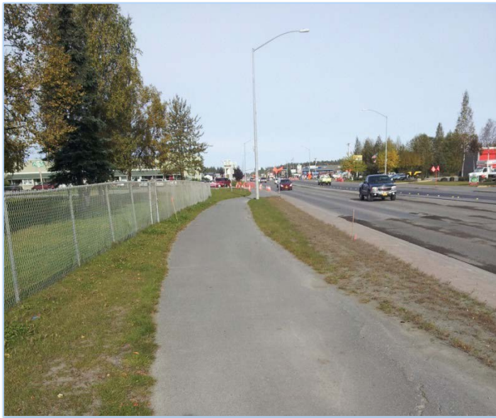
Figure 8-1 – Multi-use path adjacent to Soldotna Elementary and the Kenai Spur Highway
